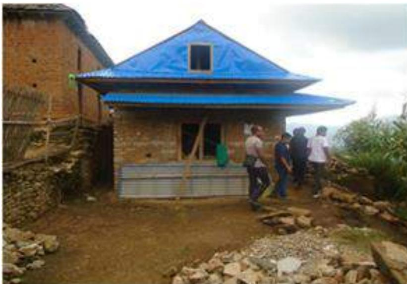
A two room house built with stone masonry and mud mortar and RCC banding in Rampur VDC, ward 7. This household have received the first and second tranches of the GoN housing reconstruction grant.
