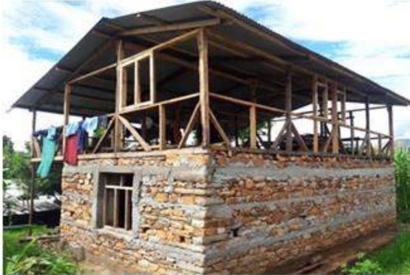
House under construction in Baideshwor Rural Municipality, Ward No. 6. This is a hybrid structure using stone masonry and mud mortar with RCC banding on the ground floor, and timber for the first floor. The household have received the first and second tranche of the GoN housing reconstruction grant.
