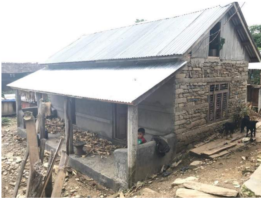
Newly constructed home in Arupokhari replicating demonstration house earthquake resilience elements.
