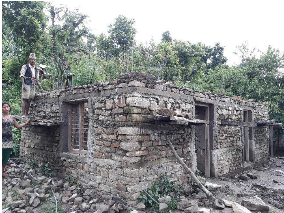
Stone masonry, Masel, Gorkha
