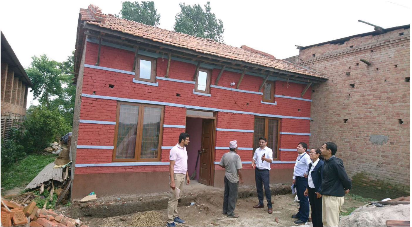
Figure 2: Newly reconstructed house of Mr. Shyam Bahadur Yando, Ward no. 3, Changunarayan Municipality, Bhaktapur, 2 storey BMM with attic; Source: HRRP, March 2020
